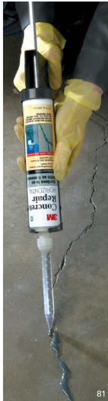
3M™ Concrete Repair 600 self-leveling flows smoothly into cleaned cracks and gaps and hardens in as little as 5 minutes.
